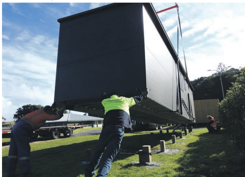
Installing the new units.
